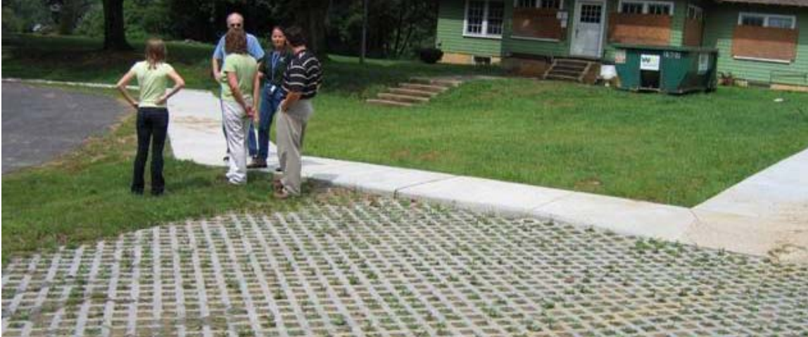
Grass pavers installed at Wong Park
